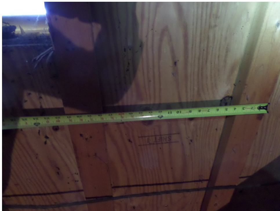
Figure 3 - Gable end truss framing with flatwise 2x4's.
